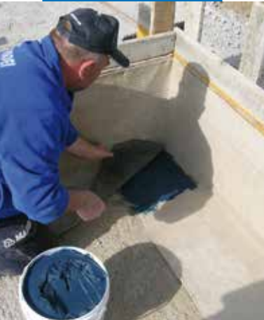
Grouting a corner of the sheet with Mapeproof Mastic
