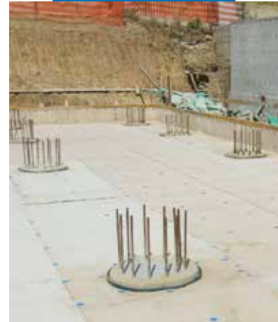
Waterproofing a foundation slab with through piling
