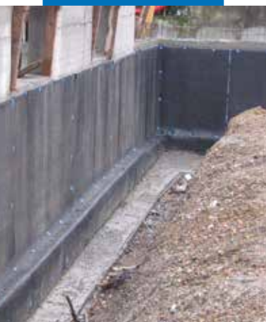
Waterproofing vertical surfaces after pouring
