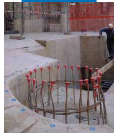
Waterproofing a top-down roof with Mapeproof
