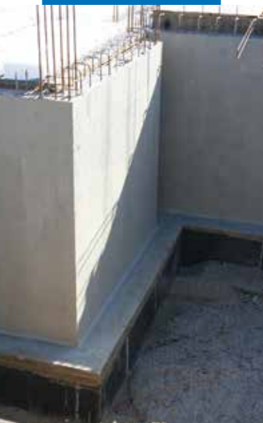
Waterproofing vertical surfaces with Mapelastic Foundation
