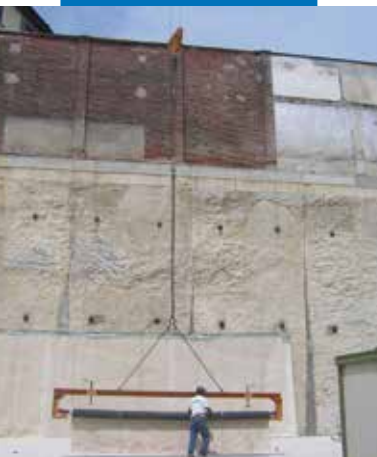
Waterproofing vertical surfaces made up of diaphragms
