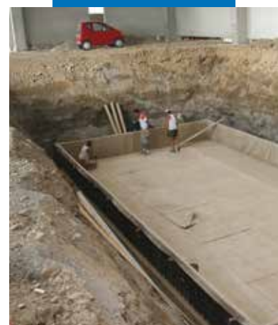
Waterproofing a horizontal surface with Mapeproof
