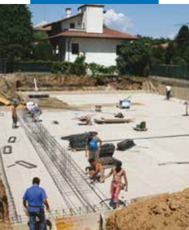
Waterproofing the foundations of a house
