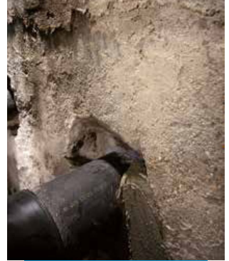
Confining Mapeproof Swell with a product of the Mapegrout line
