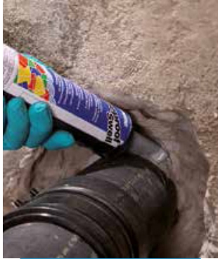
Applying Mapeproof Swell around a pipe
