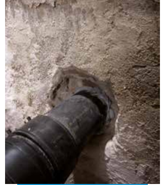
Mapeproof Swell after application
