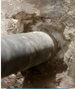
Breaking out structure around a pipe
