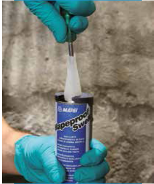
Piercing the protective membrane on the Mapeproof Swell tube
